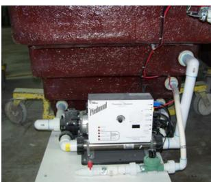
System Interface Module powered by heater. Plug Module into Heater Control Box
