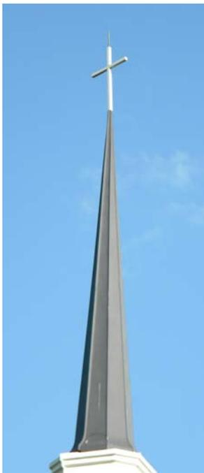
Non—PCT cross shown that rotated 30° and twisted 15° less than 6 months after installation
