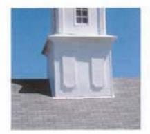
Shingle Saver is a 3/16" layer of fiberglass that is placed between the steeple base and the surface of the shingles.
